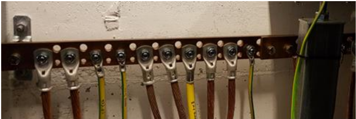
Figure 14: Main earthing bar under switchgear floor in distribution room
