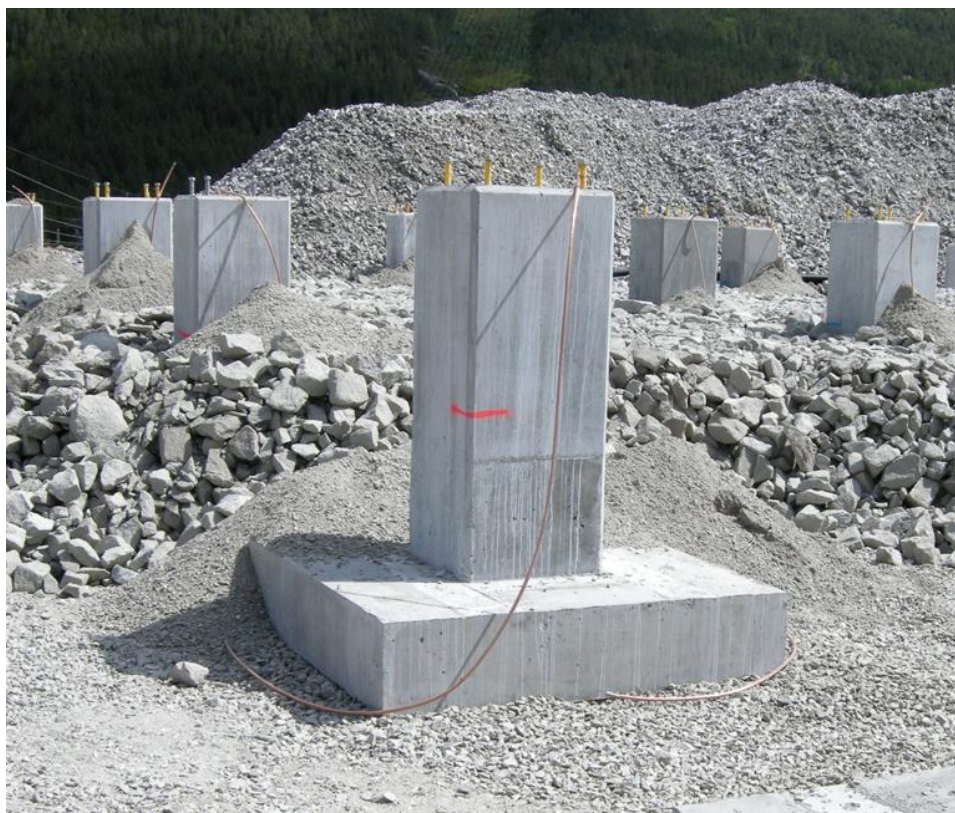
Figure 7: Example of foundation earthing
