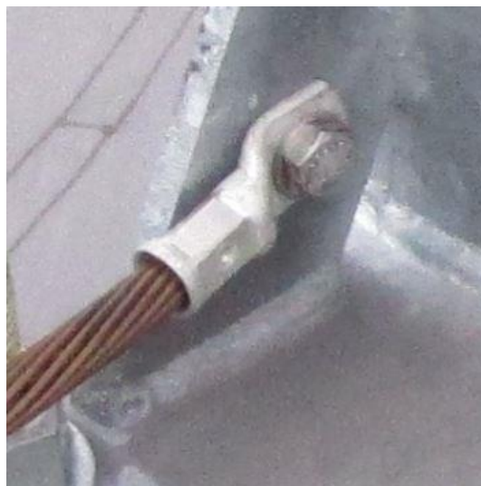
Figure 4: How to fasten cable lugs on braces
