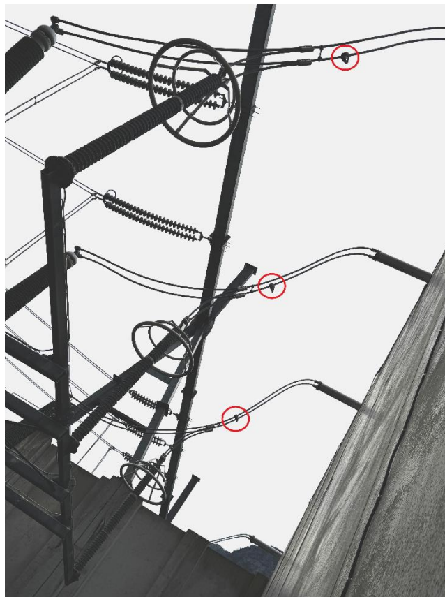
Figure 30: Brackets for attaching temporary earthing on loops towards transformers
